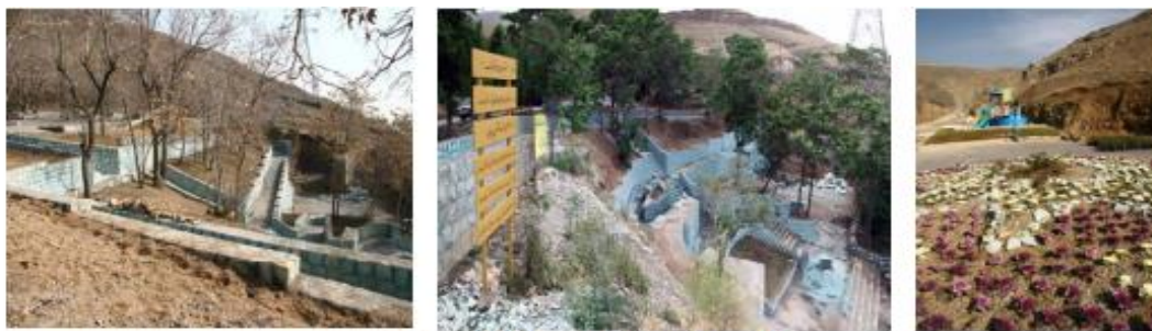
Figure 4. Pictures of the construction of Nilofer Energy Park
